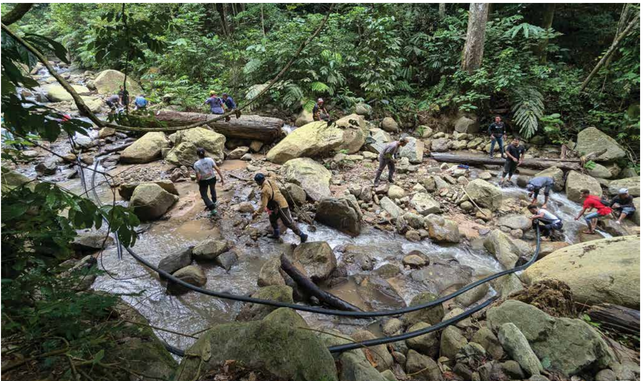
Villagers of KOA Paya Lebar worked together to repair the water pipes
