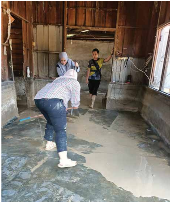
Cleaning the mud from the affected home at KOA Paya Lebar
