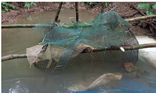
Water filter at Lata Lekah made by Paya Lebar villagers to trap fallen leaves from blocking the water pipes
